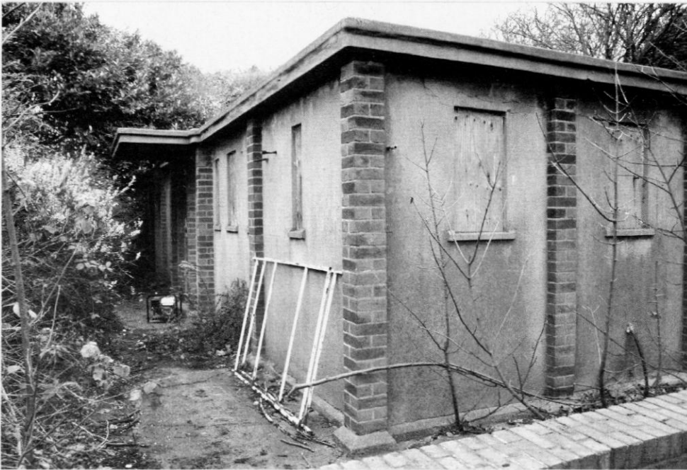
The main entrance to the Regional War Room/Group Headquarters
